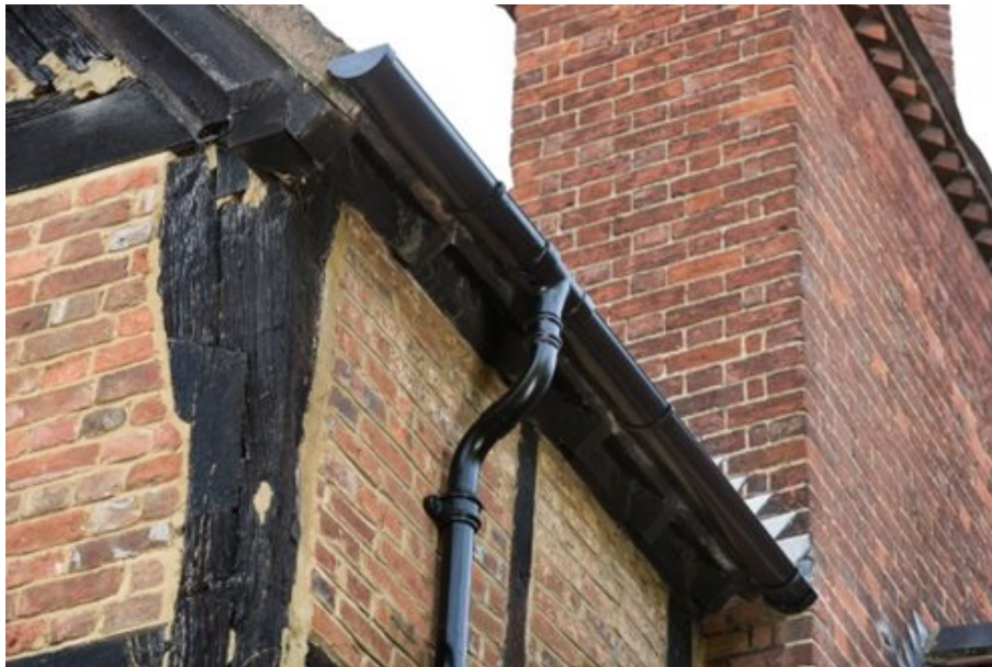
Aluminium rainwater system can be the ultimate replacement for cast iron on listed and period style properties
