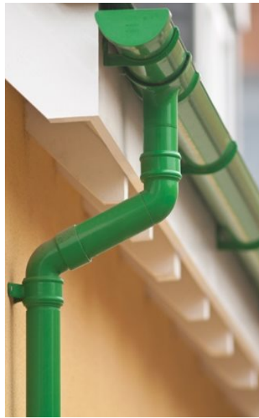
Mix of materials – aluminium gutters and downpipes installed on timber fascia and soffit
