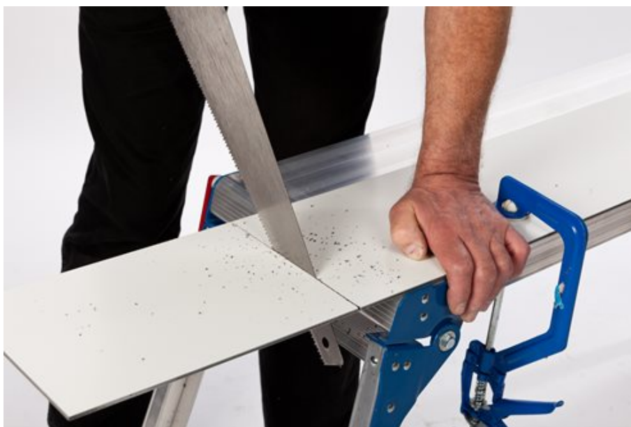
Aluminium composite fascia and soffit system can be cut and formed on site
